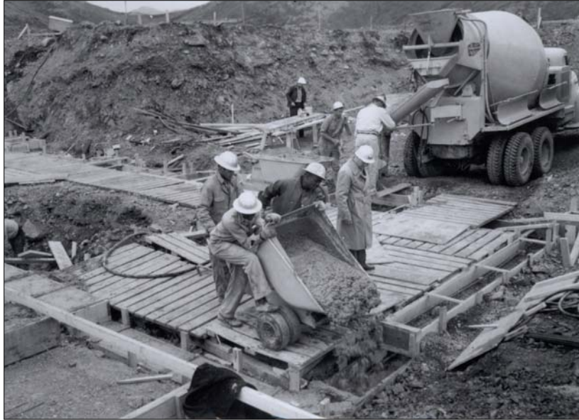
Figure 5: Construction workers pouring concrete ---Site Summit. National Archives and Records Administration. RG 77.
